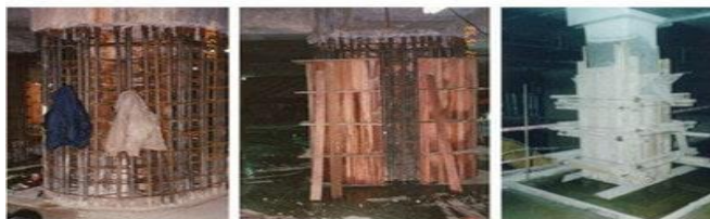
Basement steel stanchion finally encased with reinforced concrete to become permanent column
