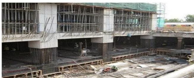
Basement steel stanchion finally encased with reinforced concrete to become permanent column
